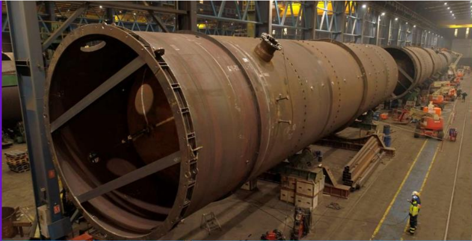
Fabrication of storage tanks by Idesa, Spain
